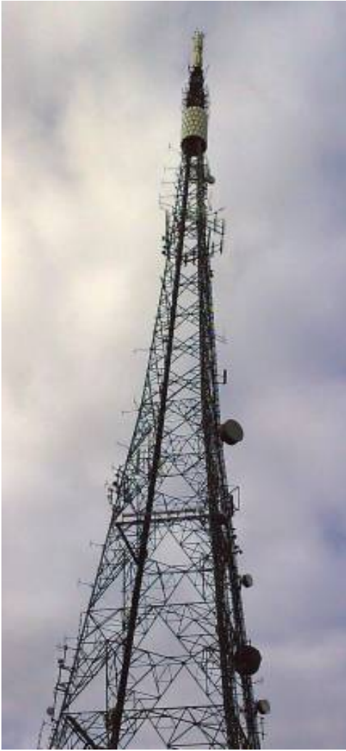
Figure 3: Craigkelly tower (left) and top section showing FM arrays (right)
