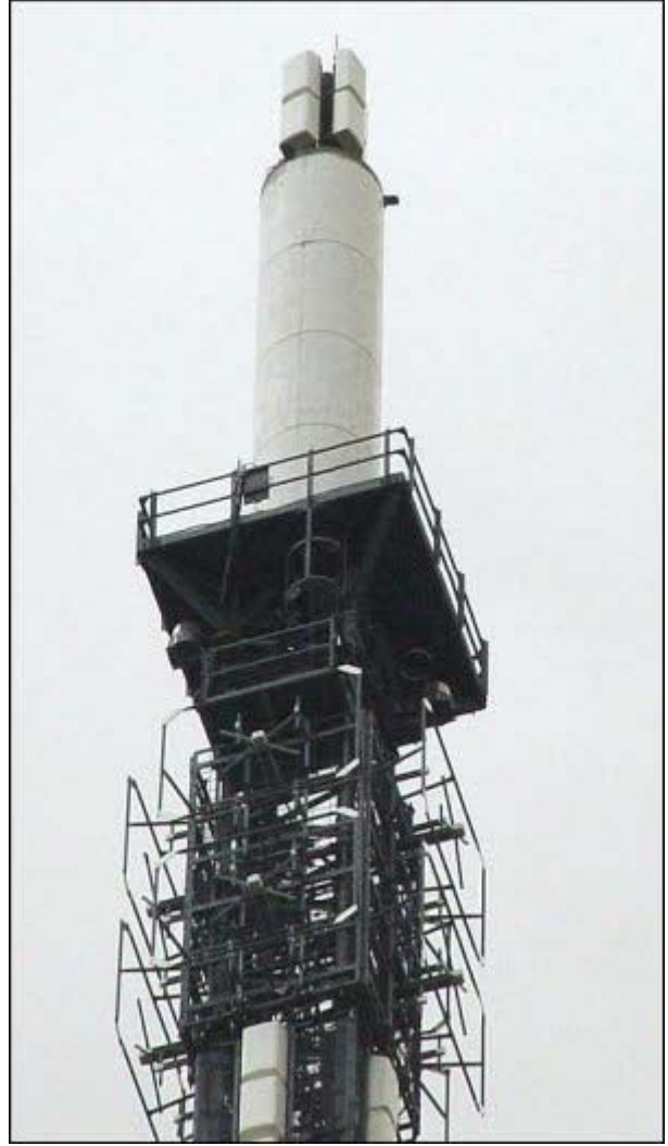
Figure 3: Craigkelly tower (left) and top section showing FM arrays (right)
